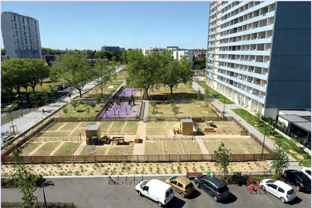
© Paul Landauer, architecte-urbaniste
